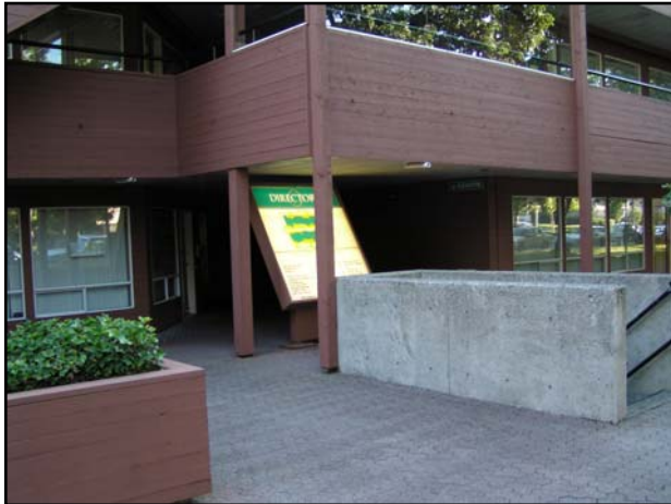
255 West 1 st Street – Elevator access
