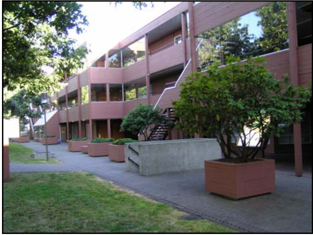
North side of 255 West 1 st Street Looking east
