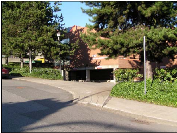
P2 Parking entrance – West side
