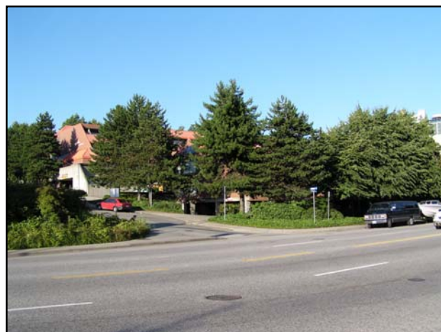
Southwest corner of 260 West Esplanade
